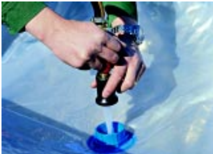
Low pressure filling: form the liner into a cube using attached adhesive tapes. High pressure filling from top or bottom: attach filling hose.
